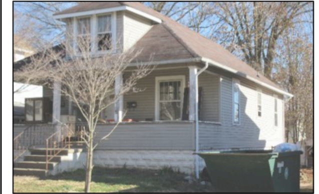
After Successful Renovation and Removal from the Building Enforcement Agency Agenda
