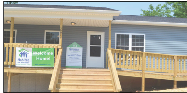
Habitat for Humanity
